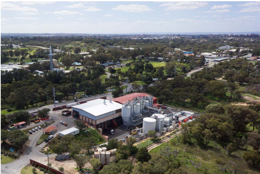
Figure 2: View of the AnaeCo™ plant facing north east, with the suburb of Shenton Park in the background.
