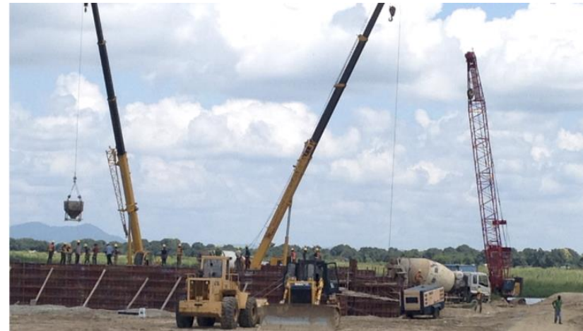
New Road and Bridge Constructions on route to Epanko
