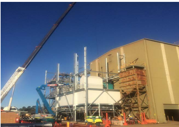
Figure 2: Coronastat being installed at the Picton mineral separation plant
