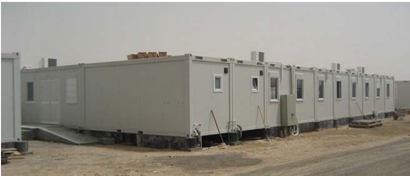
Modular Offices and Camp (example)
