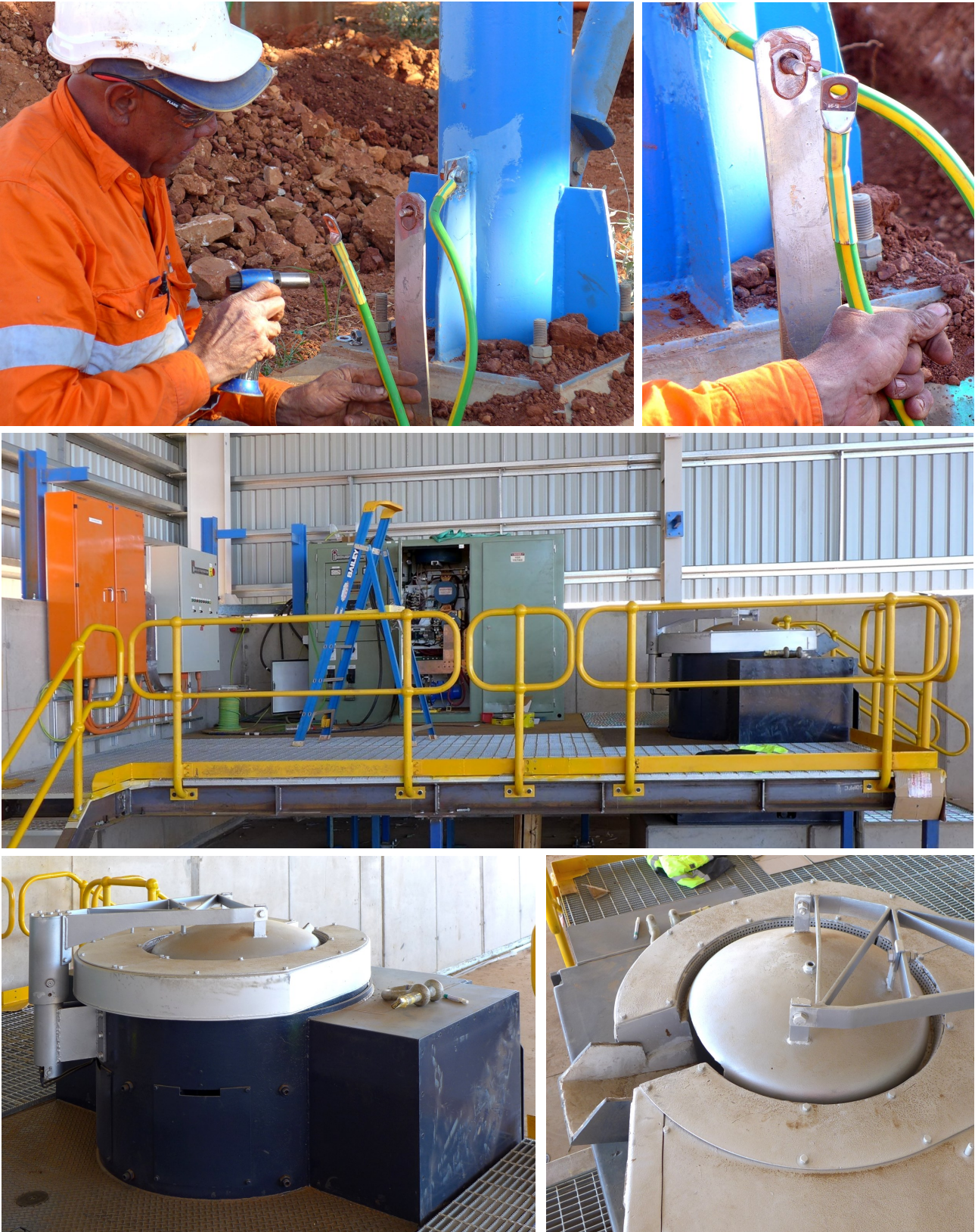
Figure 10: Electric Furnace installation is nearing completion.
