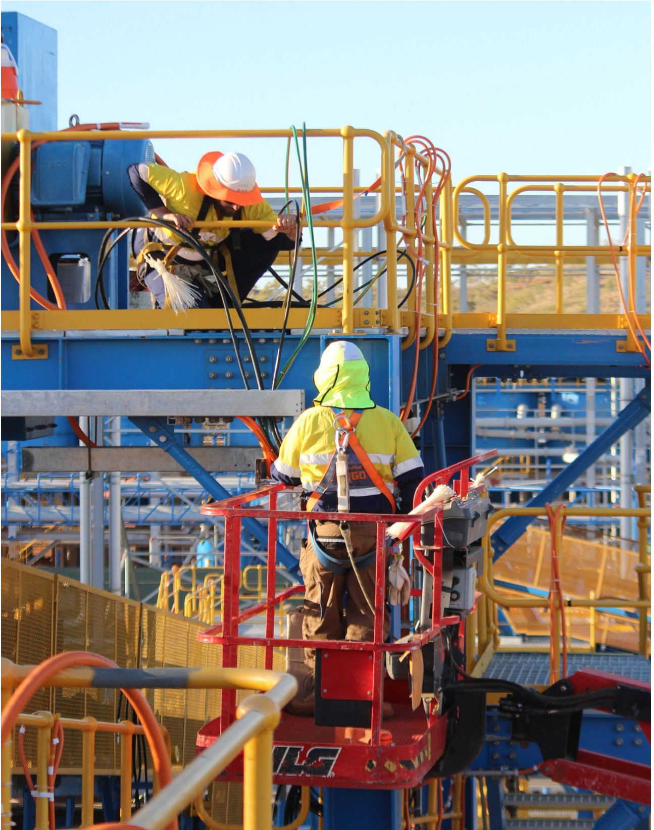
Figure 3: Cable being installed.
