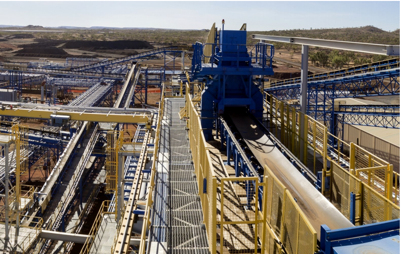
Figure 6: Various views of the Process Plant; (with ROM in background (top) and crushed ore stockpiles in background (bottom))
