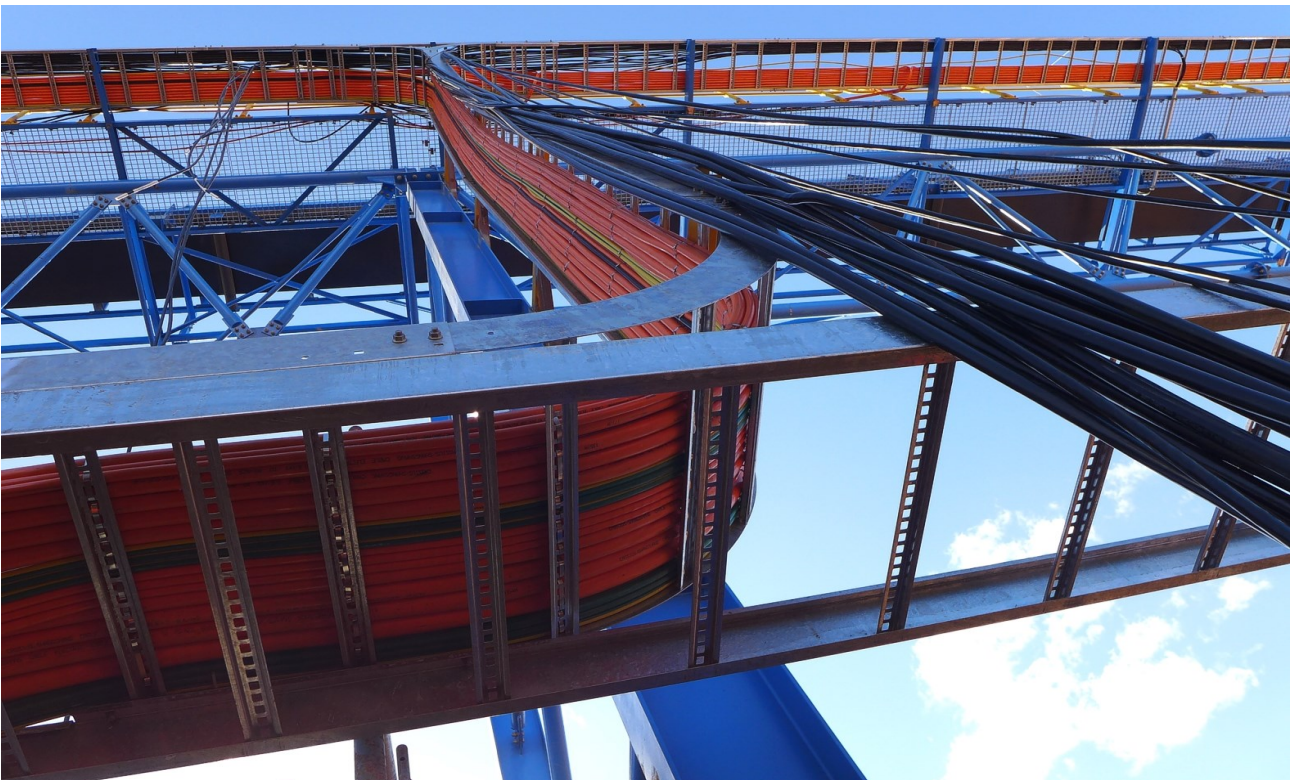
Figure 7: Over 120 electrical contractors are involved in cable and associated infrastructure installation.
