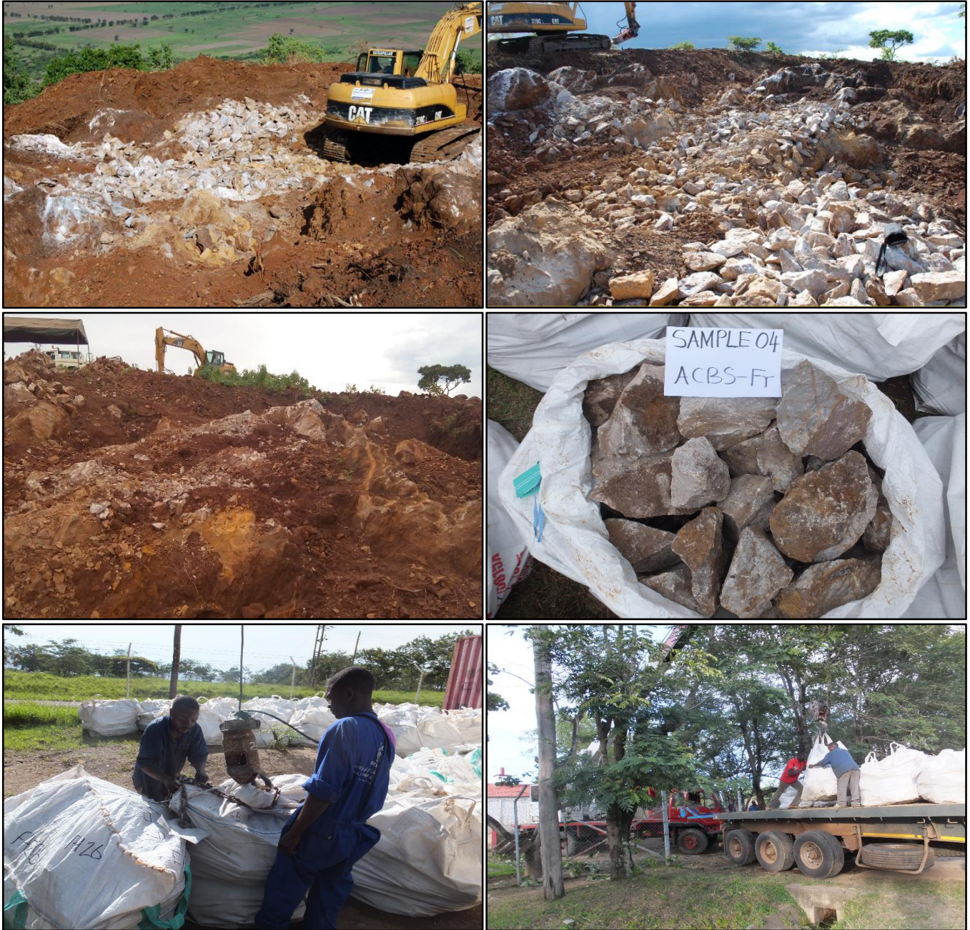
Figure 2: Showing the 3 pits being excavated (A – top left, B – top right, C – middle left) and an example of a 1 tonne bulk sample from Area A (middle right). Collection and cartage of the bulk samples is shown at the bottom.
