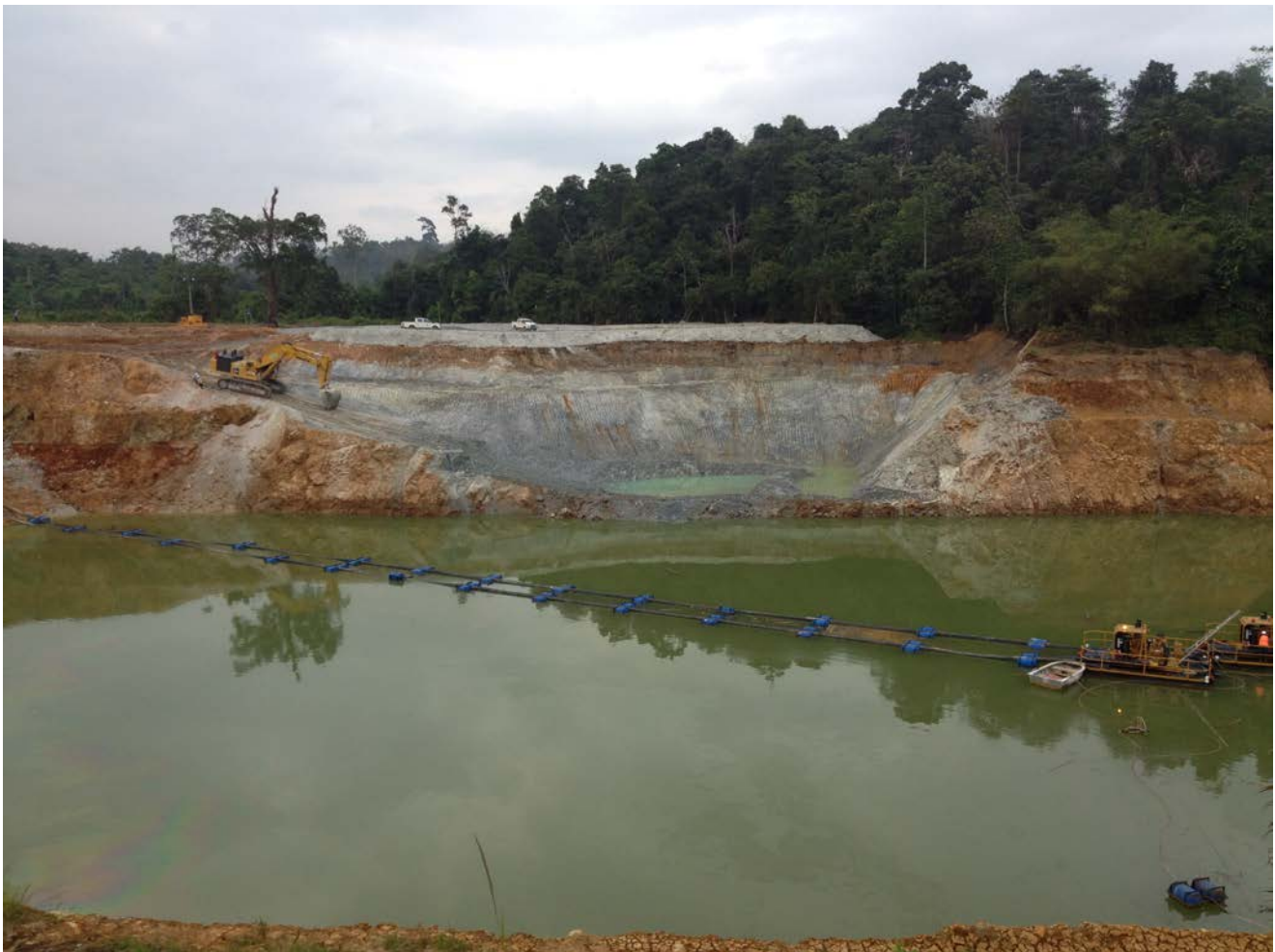
Figure 1. Belinau pit dewatering with portal access works in the background
