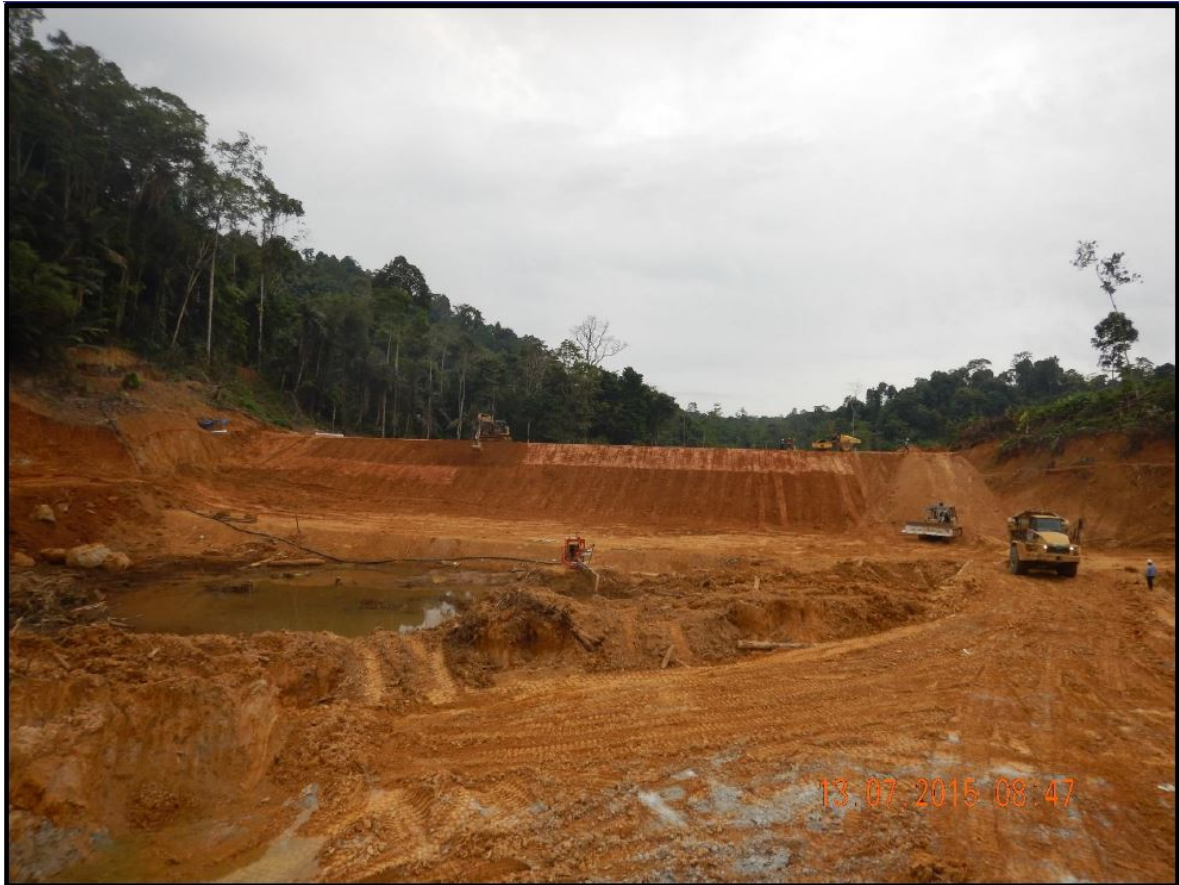
Figure 2. Construction of the temporary tailings storage facility (now complete)
