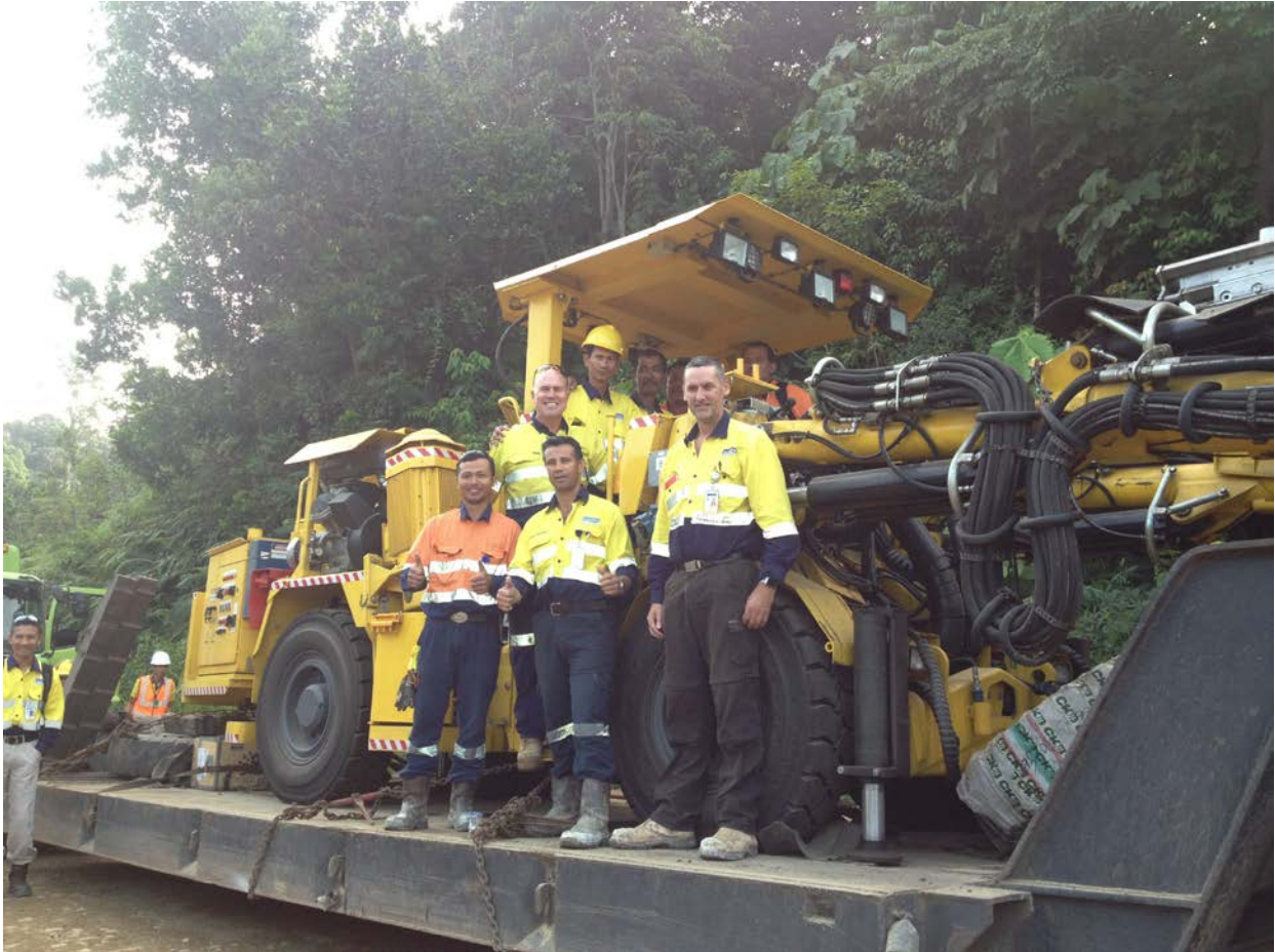
Figure 6. Jumbo underground drill on site with operations team
