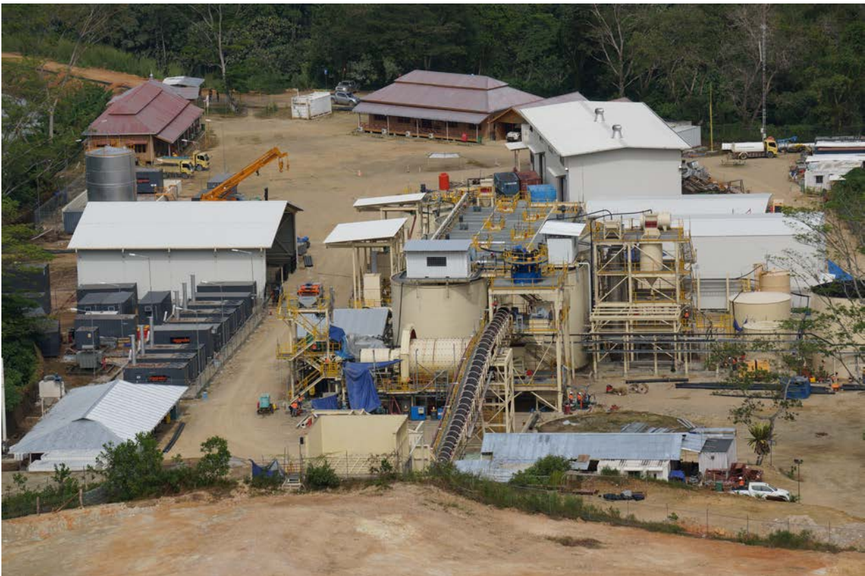
Figure 5. CIL plant with edge of ROM pad in the foreground
