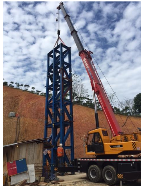
Figure 3: Installation of completed headframe
