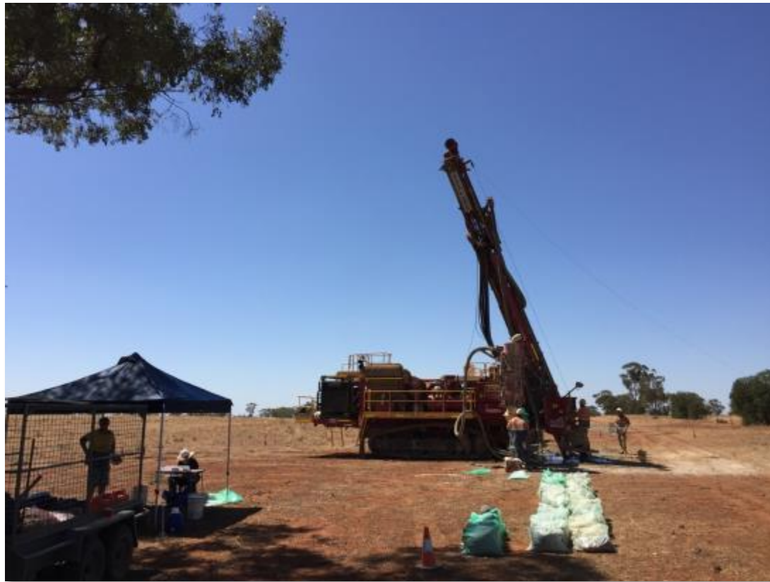
RC Drilling | Collerina March 2015
