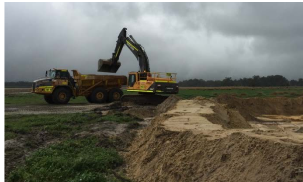
Figure 5: Mine Feed Unit earthworks at Keysbrook
