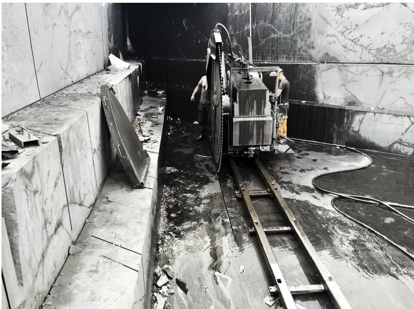
Figure 1. Trial mining underway in high grade graphite ore at Talga's 100% owned Vittangi project in Sweden.
