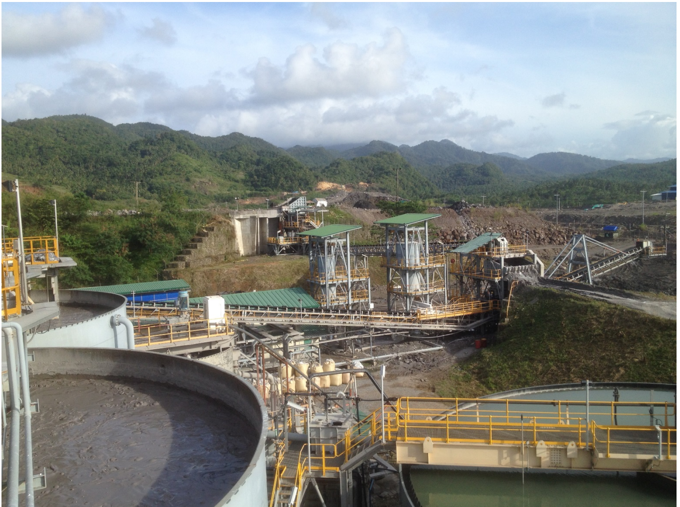
Figure 3: View of the Siana processing plant with thickener and CIL tank in foreground
