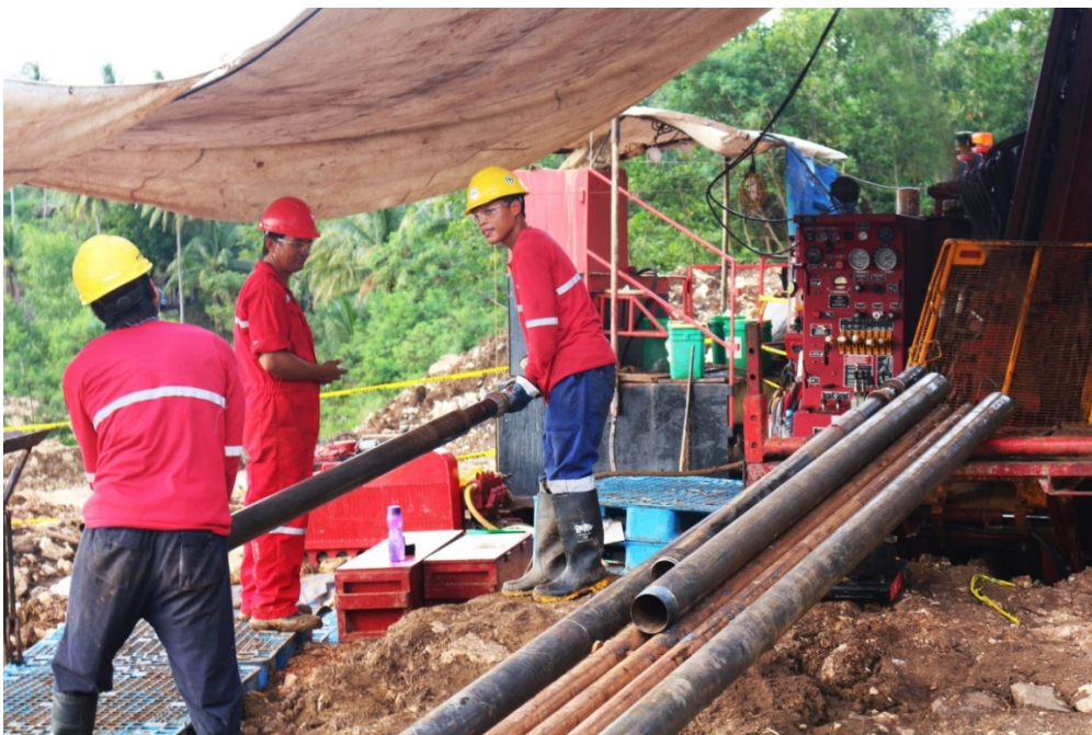
Figure 6: Geotechnical diamond drilling underway at the Eastern pit wall
