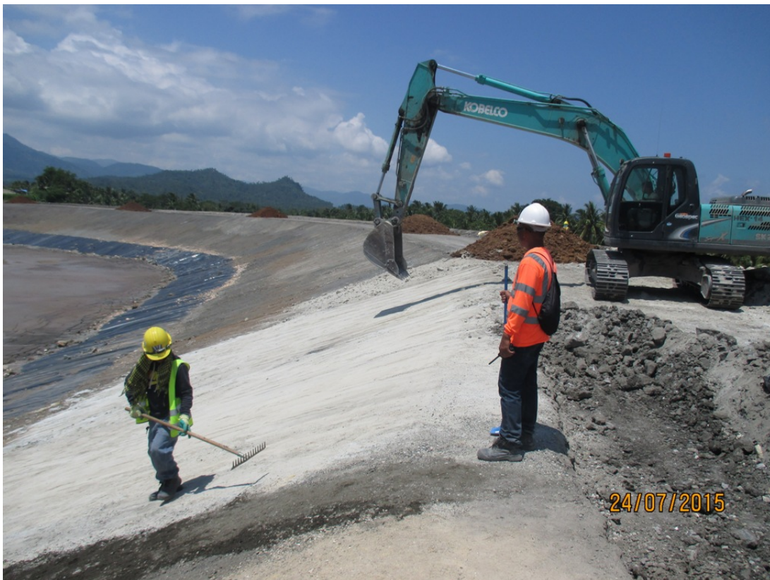
Figure 4: HDPE Tailings Storage Facility construction
