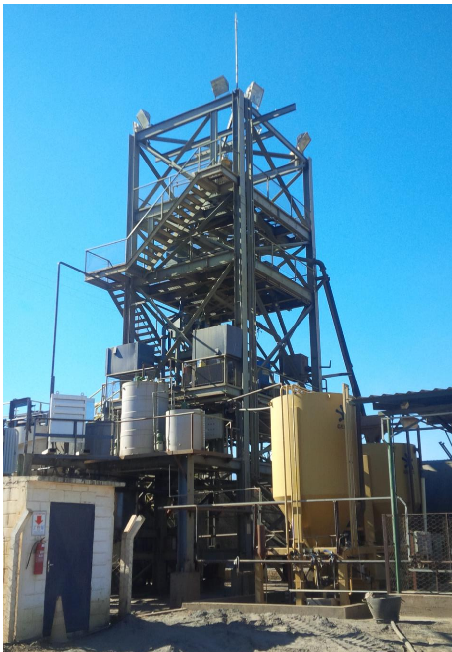
Stacked celled flotation (tanks and control systems seen in centre left of picture) installed in Premier process plant
