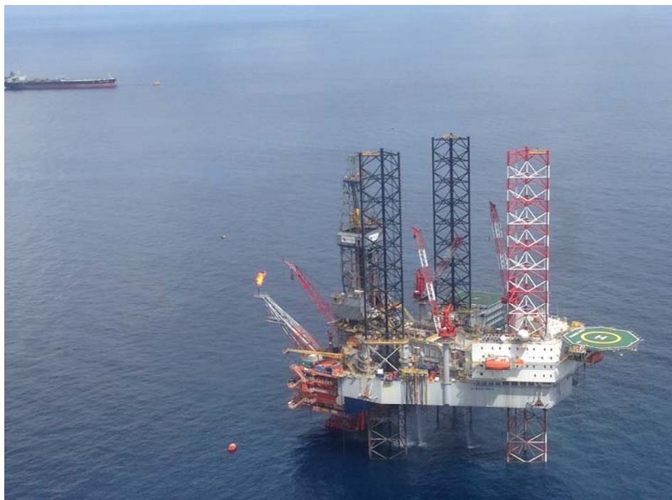
Platform with Manora Princess FPSO in background
