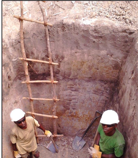
Figure 3. Typical trench dug over primary VTEM anomaly – notice the graphitic soil and bedrock
