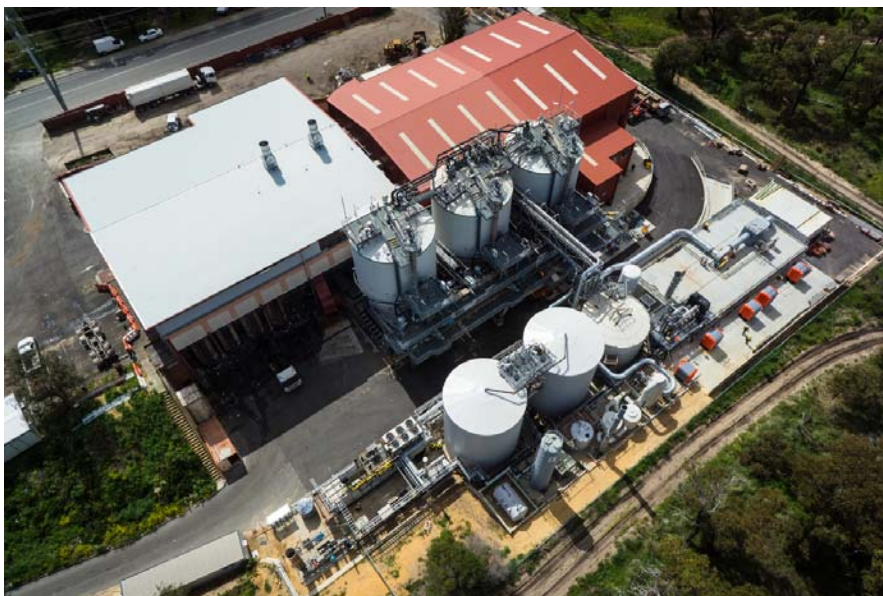
Figure 1 : AnaeCo™ AWT Plant at WMRC JFR McGeough Resource Recovery Facility, Shenton Park, Western Australia
