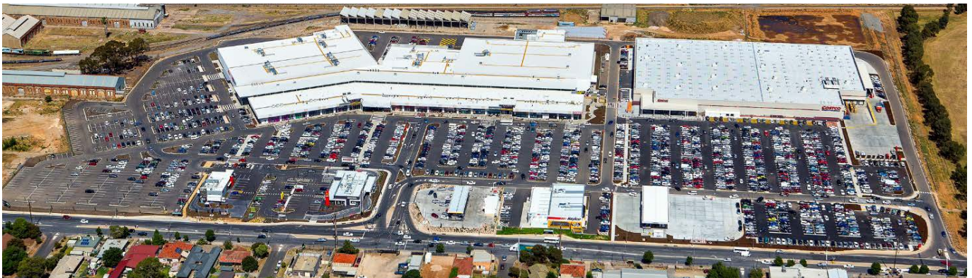
Churchill Centre North as at November 2014
