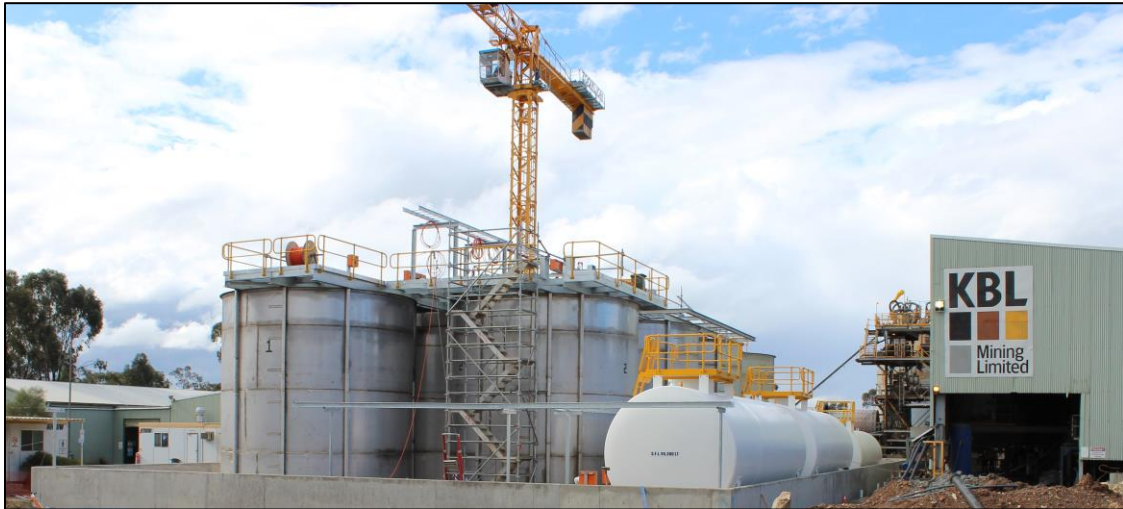
Photograph 5: CIL construction progress
