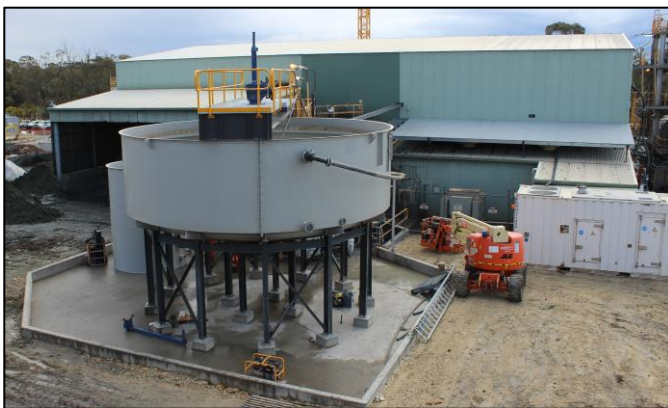
Photograph 3: 8 metre Thickener, Reagents storage
