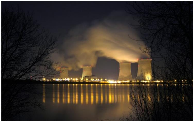
The Electricite de France (EDF) nuclear power station of Cattenom near Thionville, Eastern France, is seen at night February 8, 2012. Vincent Kessler/Reuters
