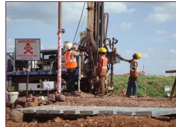
Drilling underway at Kuja
