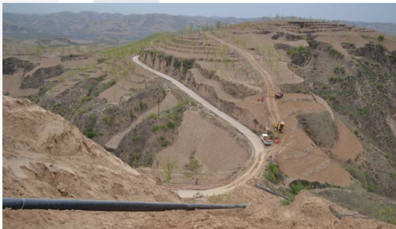
SGE gathering lines being installed
