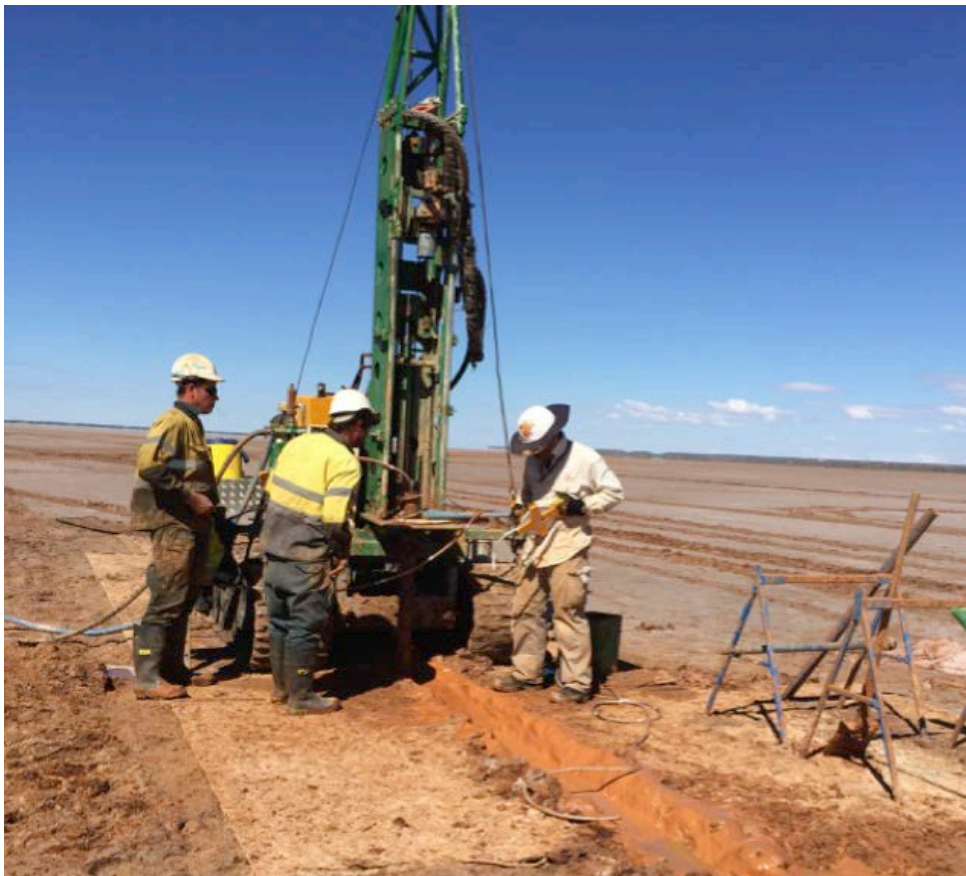
Figure 1 – Drill Rig in Operation
