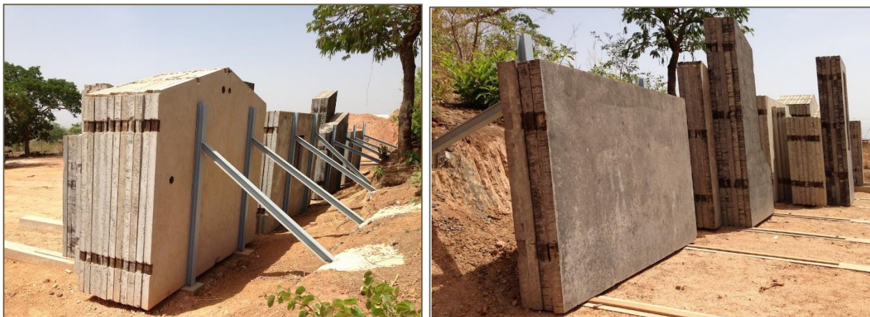
Picture 1: Banfora Gold Project | Locally Fabricated Panels for Resettlement Houses
