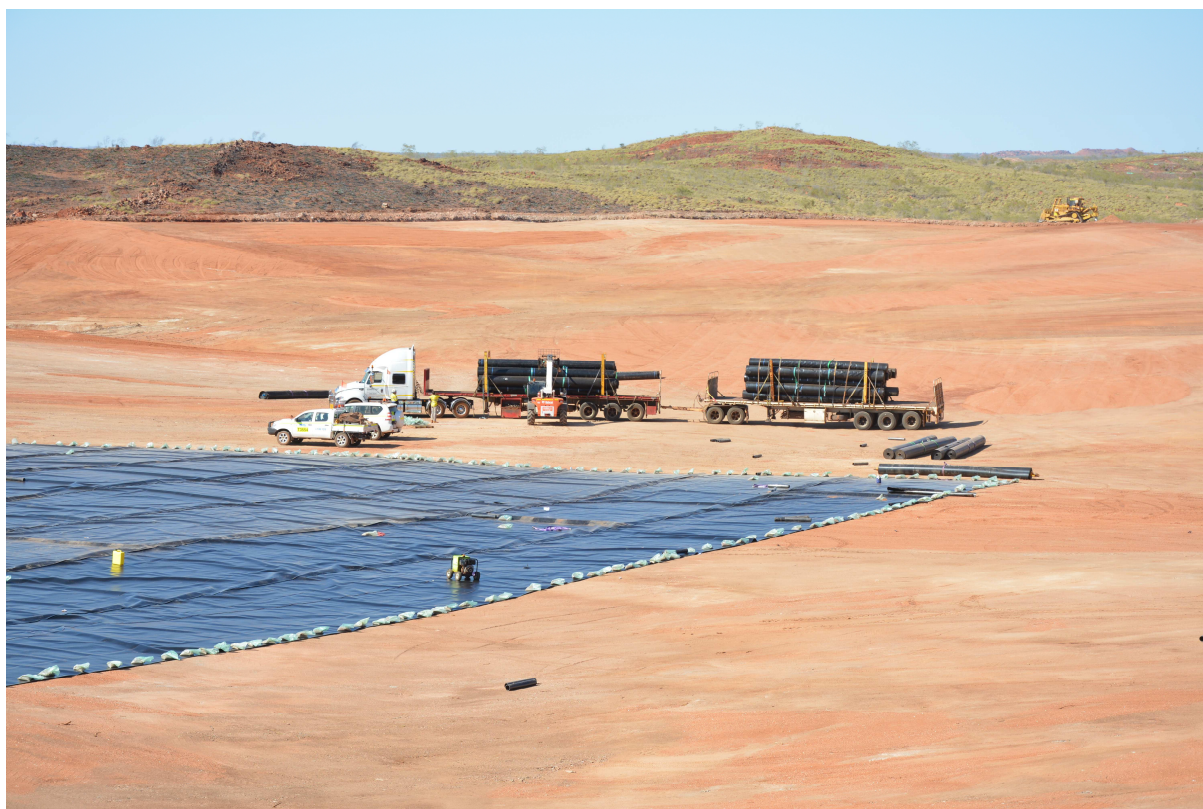
Tabba Tabba installation of liner for tailings storage facility September 2015
