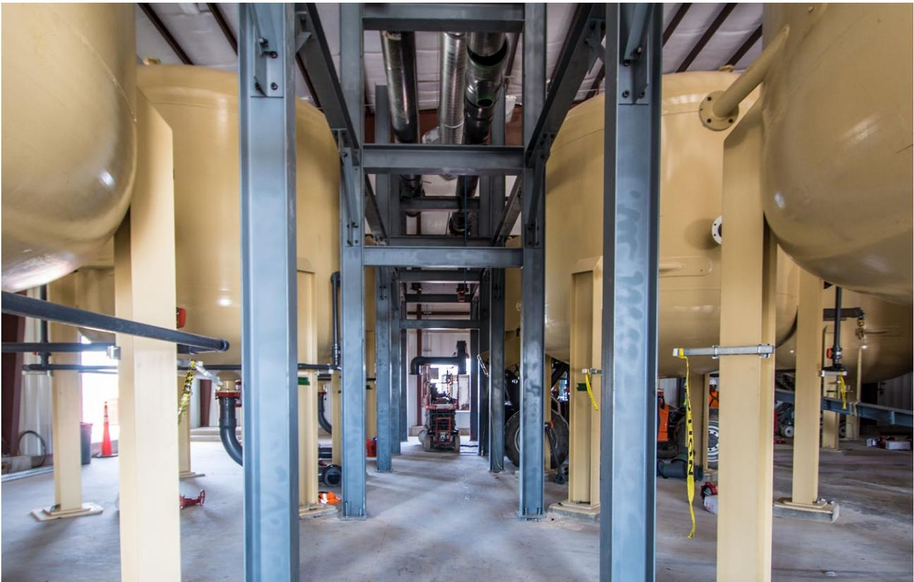
Figure 4: Completed Ion Exchange Columns within the CPP, Wyoming USA
