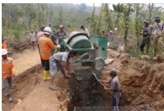
Image 1: Concreting activities relating to suspension bridge at Sindang Jaya
