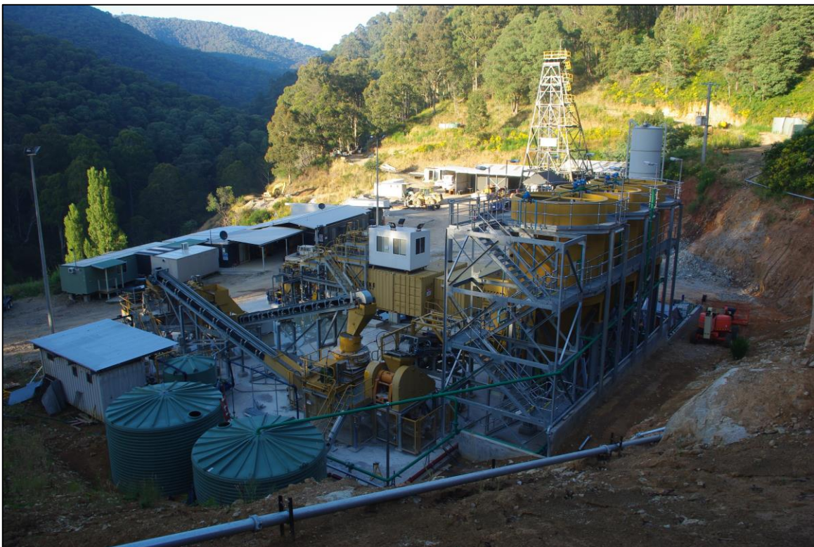
Picture 1: Morning Star process plant and mine offices.
