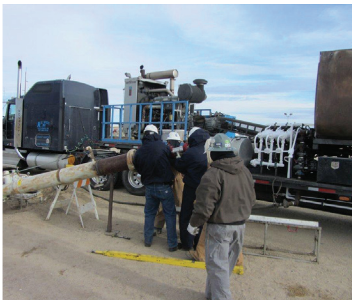
Intelligent pigs being inserted into the Grieve Oil pipeline
