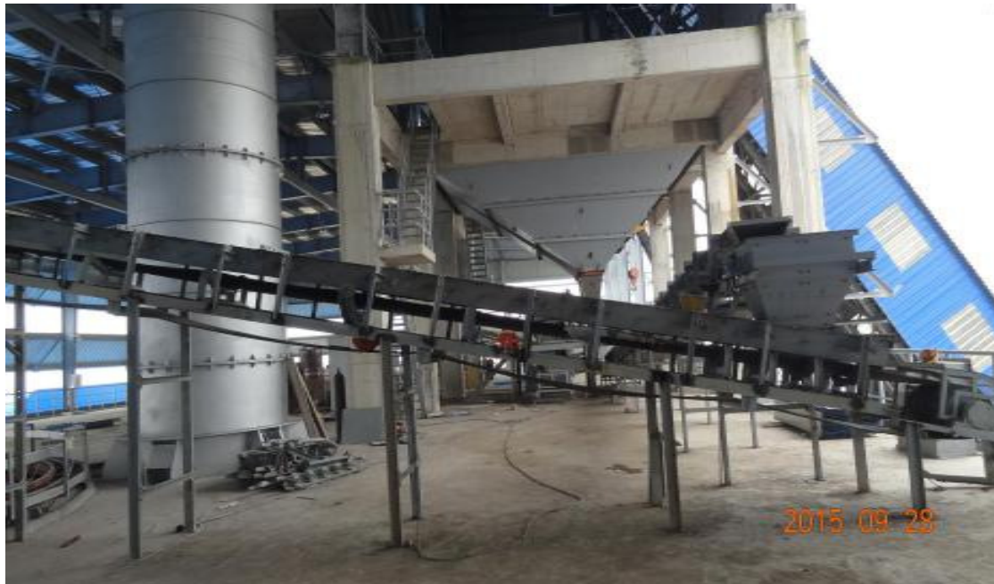
B05 Belt Conveyor system installation
