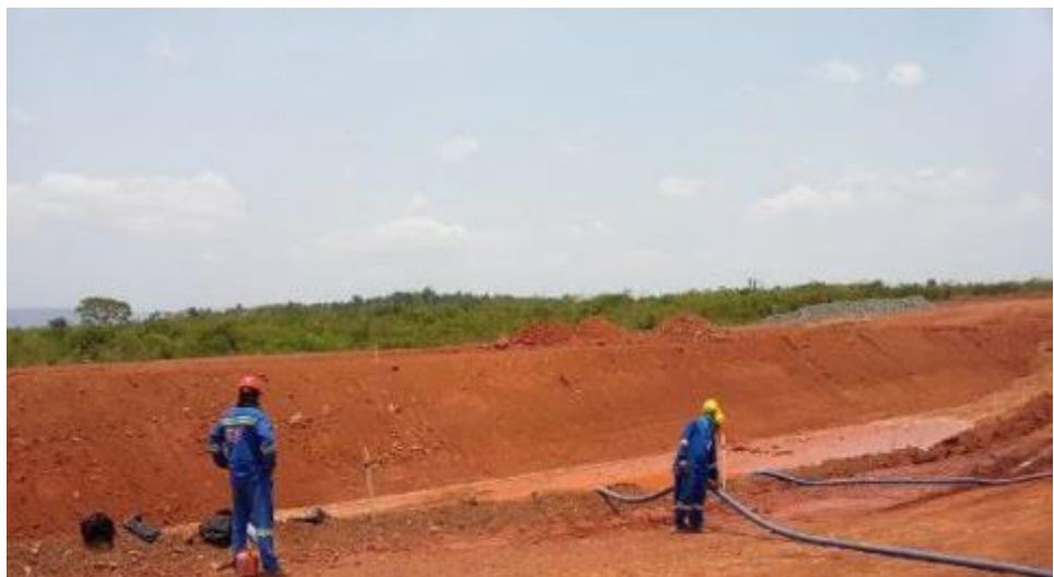
Earthworks continue to raise the crest of the dam wall
