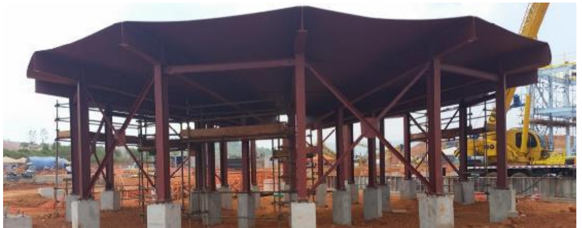
Concentrate Thickener fabrication in progress
