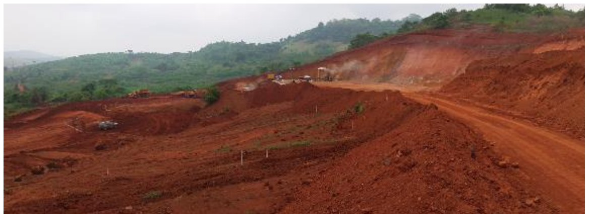
Establishment of mining benches - Antas Stage One
