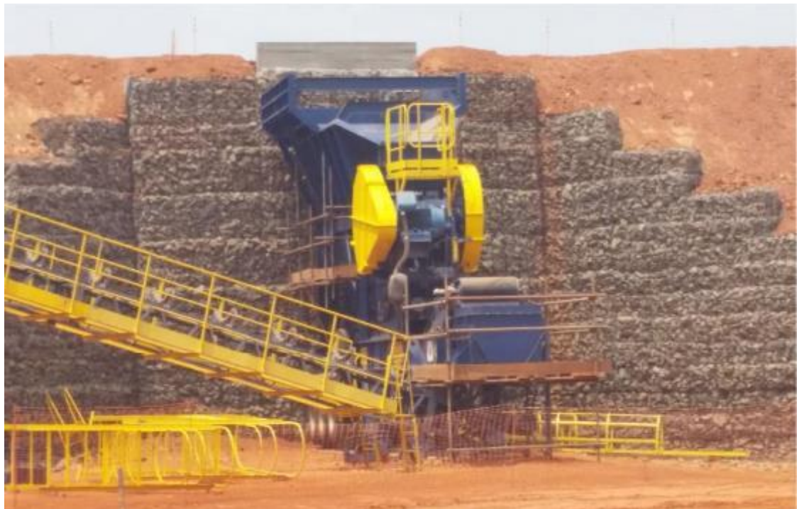
Earthworks associated with the initial ROM Pad construction are complete and the retaining wall erected. The jaw crusher is installed below the tip head, awaiting only the feed hopper, grizzly and electric
