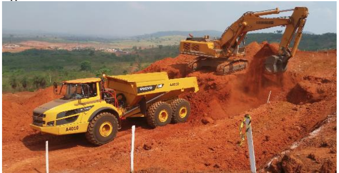
First loads - Volvo A40F and R964 excavator
