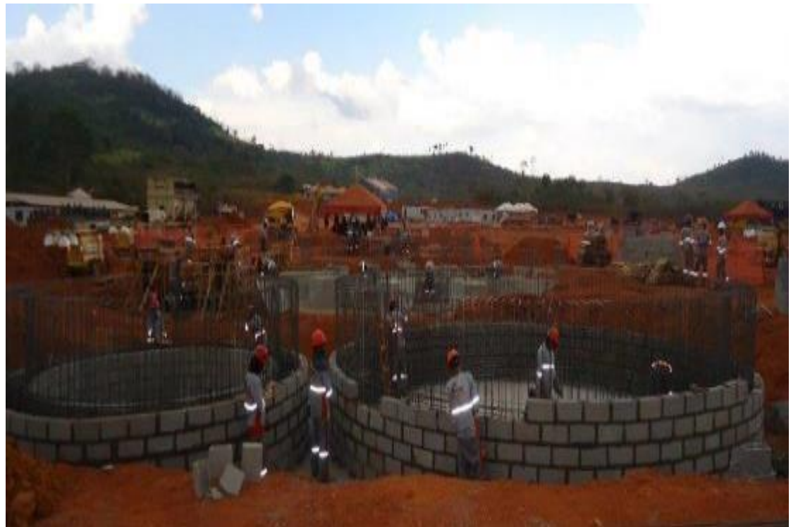
Foundations being prepared for process water and raw water tanks
