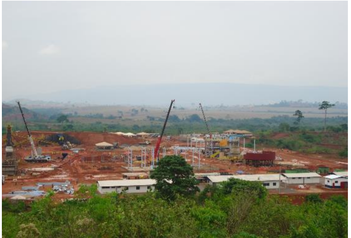
Overview of construction activities around the beneficiation plant
