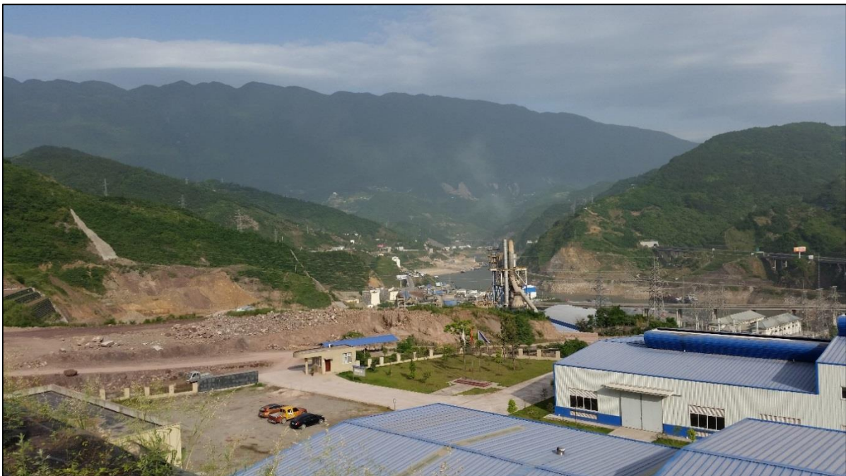
Figure 15. Xingshan proposed graphite plant site. Hydro-electric sub-station (right centre) and port loading facilities (centre).
