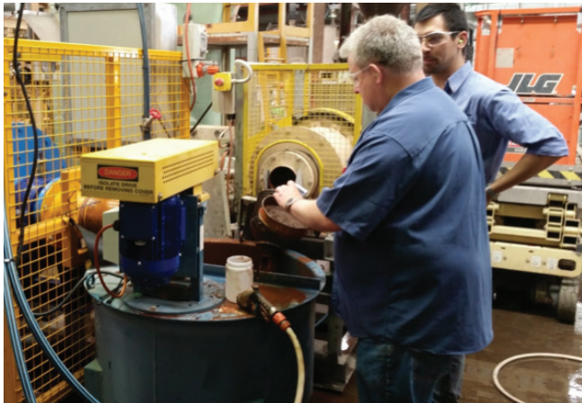
Figure 8: Greg Henderson, AMEC FW (foreground) and Roy Gordon, Peak Resources, commissioning grinding circuit at ALS.
