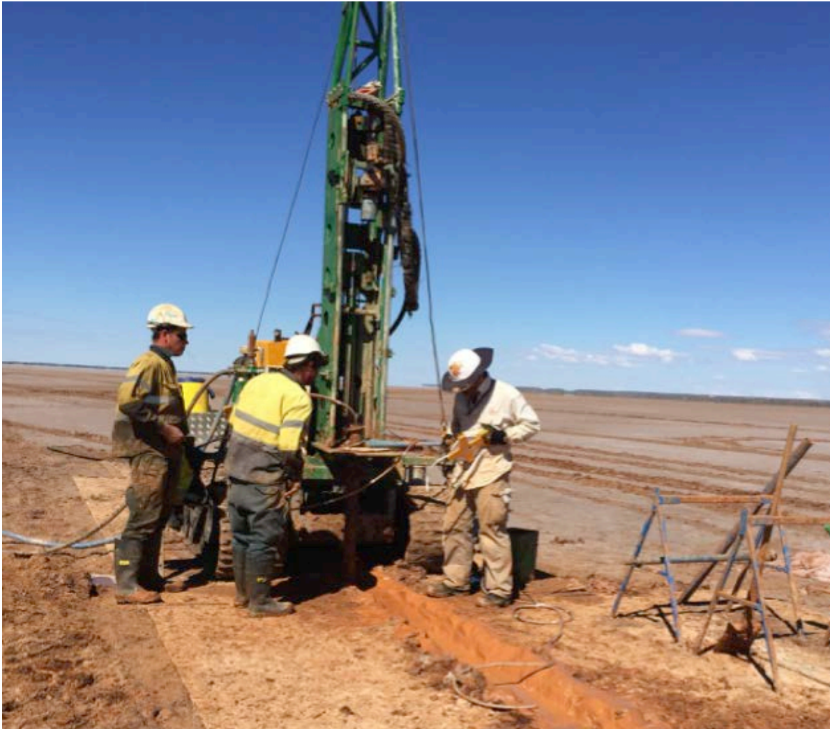
Figure 3: Drill Rig in Operation
