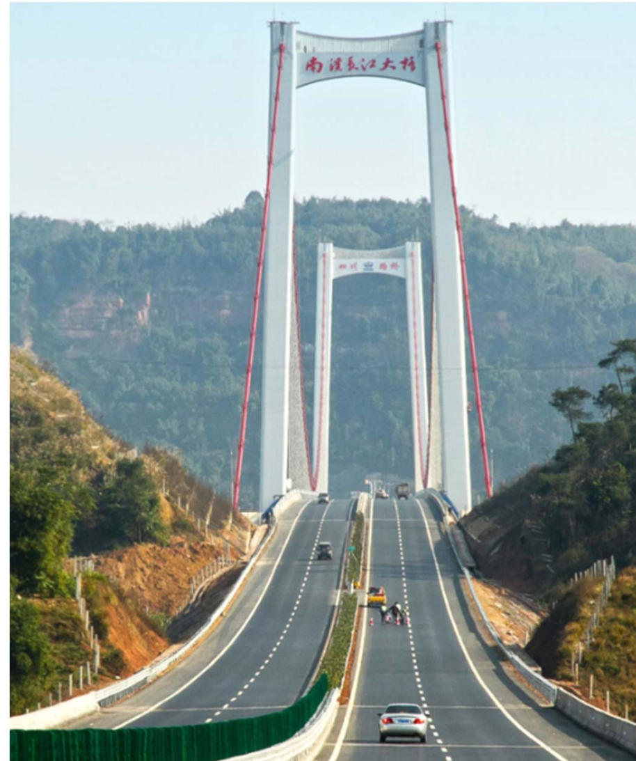
Yibin-Luzhou Highway built by SRIG
