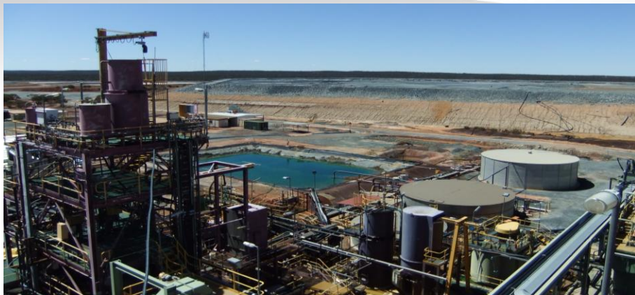
Mill with tailings dam in background
