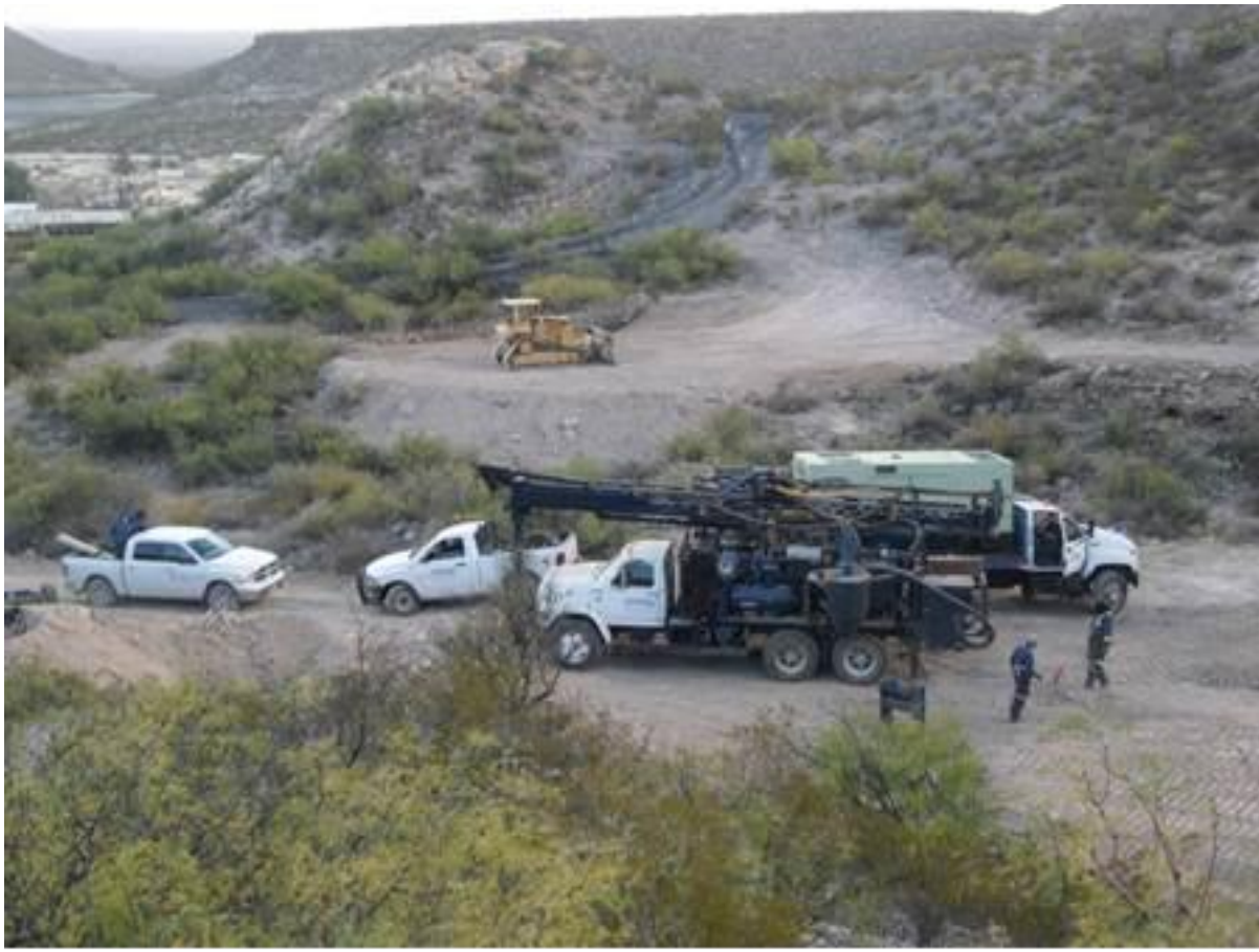
Figure 5. View across to the Plomosas site village (top left) showing the Schramm RC rig about to set up on the first surface drillhole for Tres Amigos.
