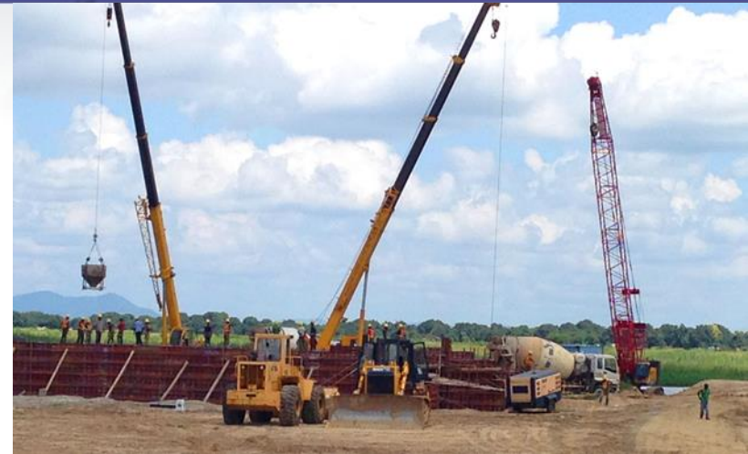
New Road and Bridge Constructions on route to Epanko
