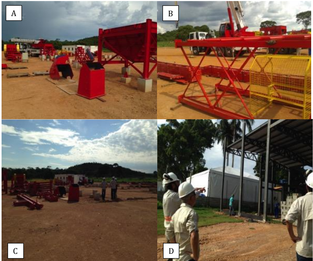
Figure 2. A. Crushing circuit being installed on foundations. B & C. Delivery of the crushing circuit. D. Construction of the mine and plant workshop.
