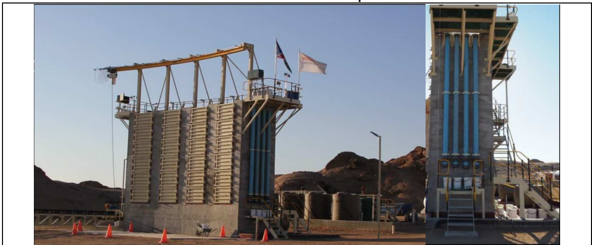
Figure 13.23 Cribs and Columns Setup
