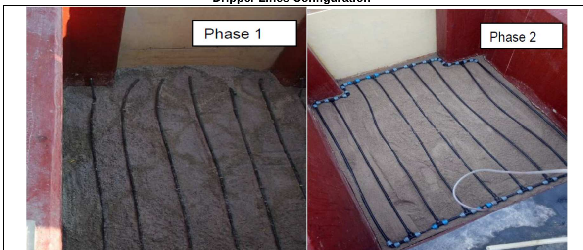
Figure 13.28 Dripper Lines Configuration
