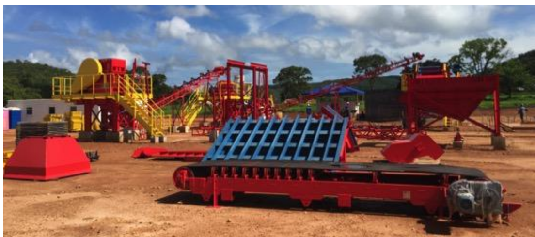
Figure 3. Construction of the Cascavel Plant.
