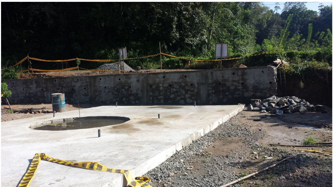
Shaft H at Aluketiya - Headframe construction will commence in February 2016
