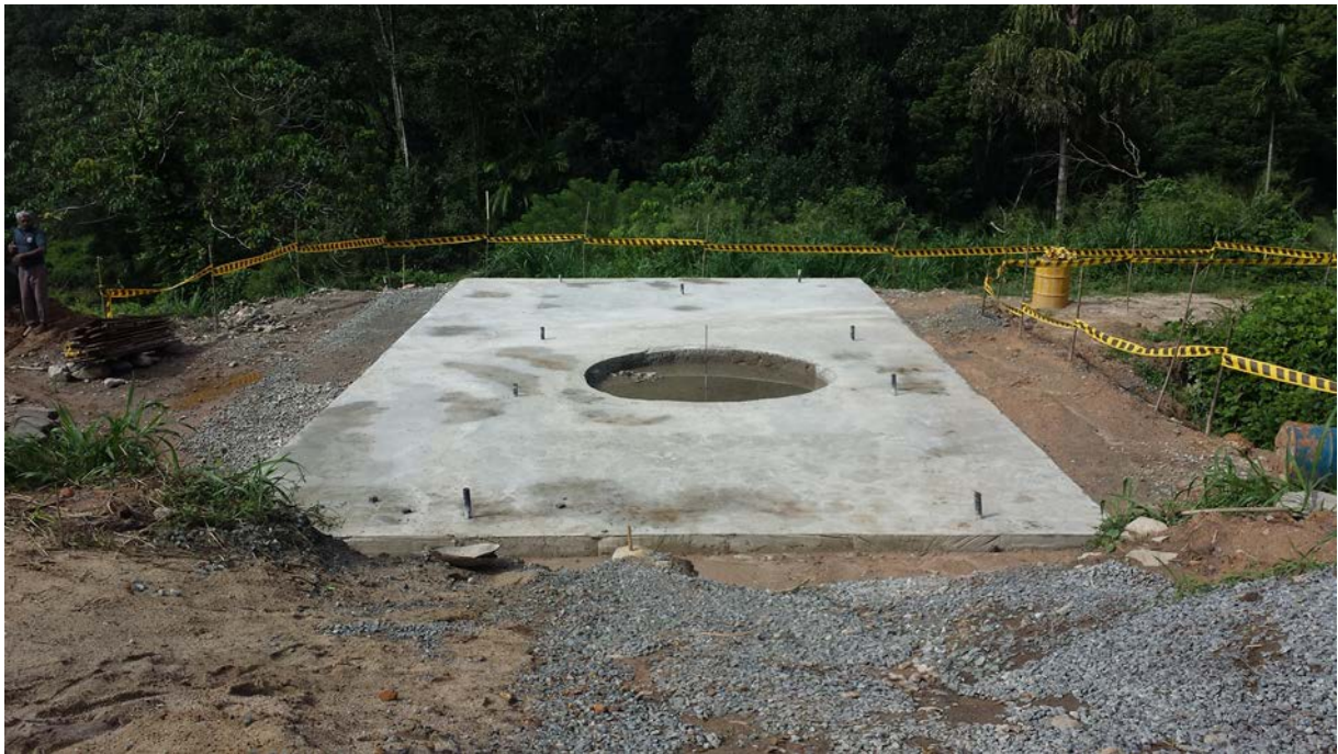
Concrete pad completed for Shaft H at Aluketiya.
