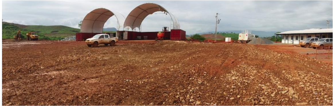
Mobile equipment workshops and mining offices now operational
