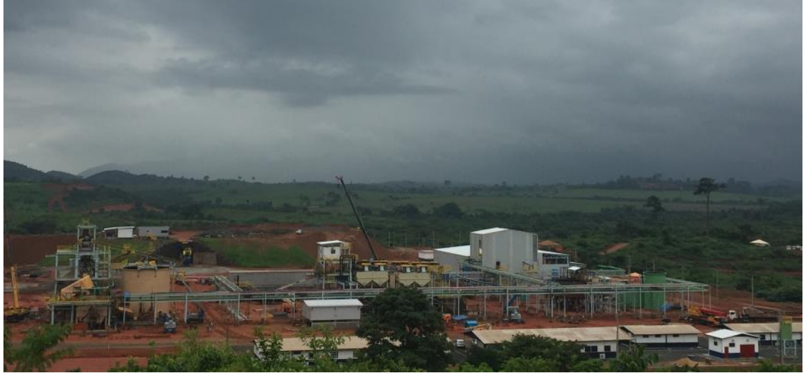
View of the beneficiation plant – construction at an advanced stage
