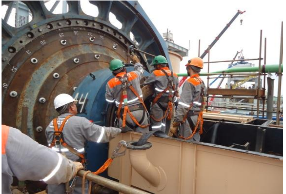
Torquing of trunnion head bolts on Metso ball mill
