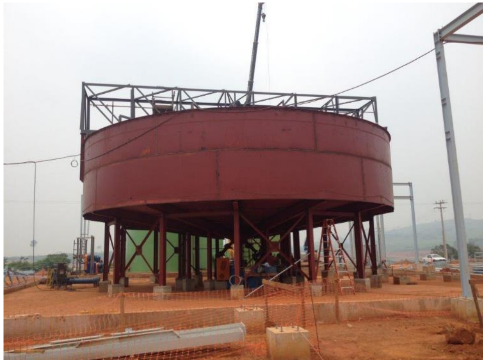
Concentrate thickener installation at an advanced stage
