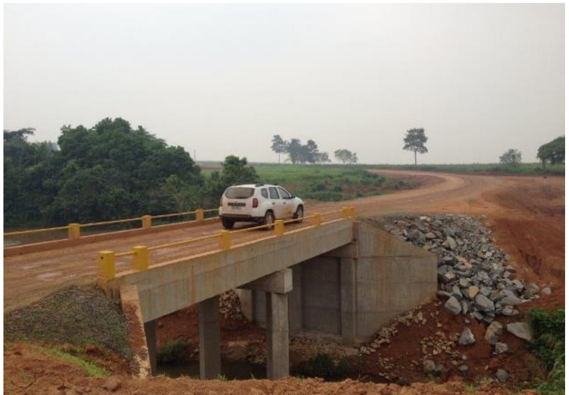
Mine access road including construction of two bridges completed
