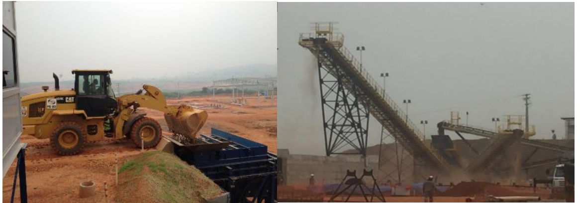
Crushing section is now operational
