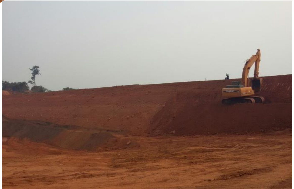
Finishing of tailings dam wall slope faces
