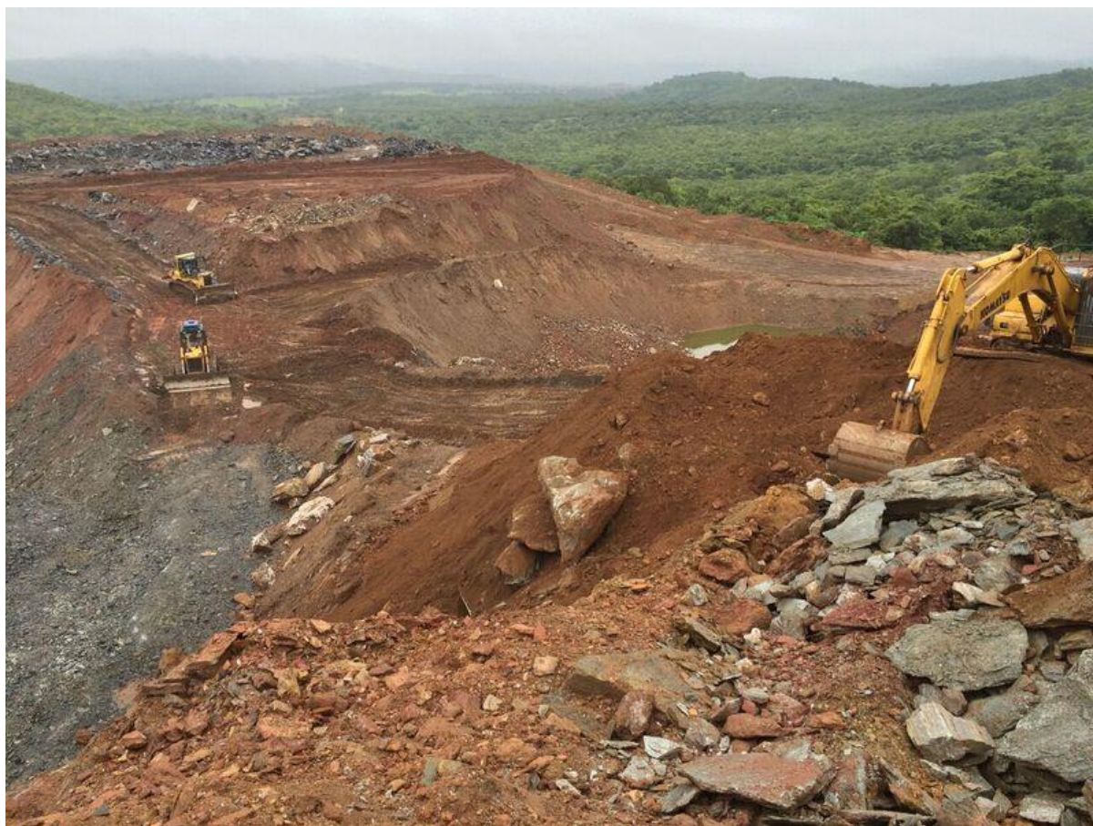
Creation of the new “Skyway” at Premier to reduce haulage distance
