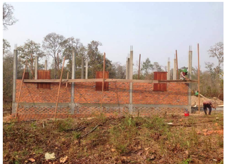
Photo Two | Ongoing construction
