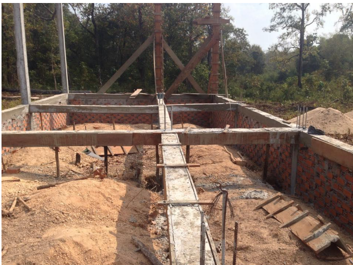
Photo One | Construction commences
