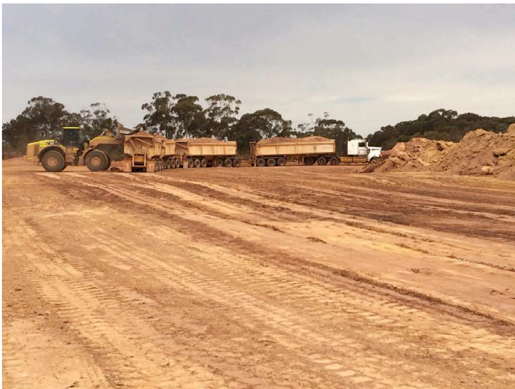
Figure 2: Haulage truck being loaded at Castlereagh ore pad.
