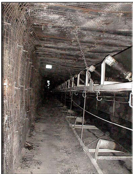
Modern Roof Bolted Coal Mine Roadway
