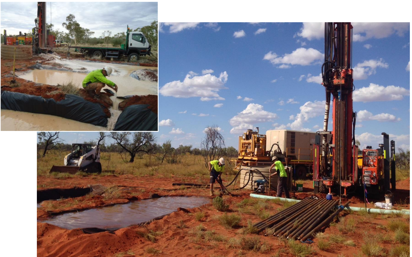
Figures 11 & 12 – LD Process Water Exploration and V-Notch Flow Testing (inset)
