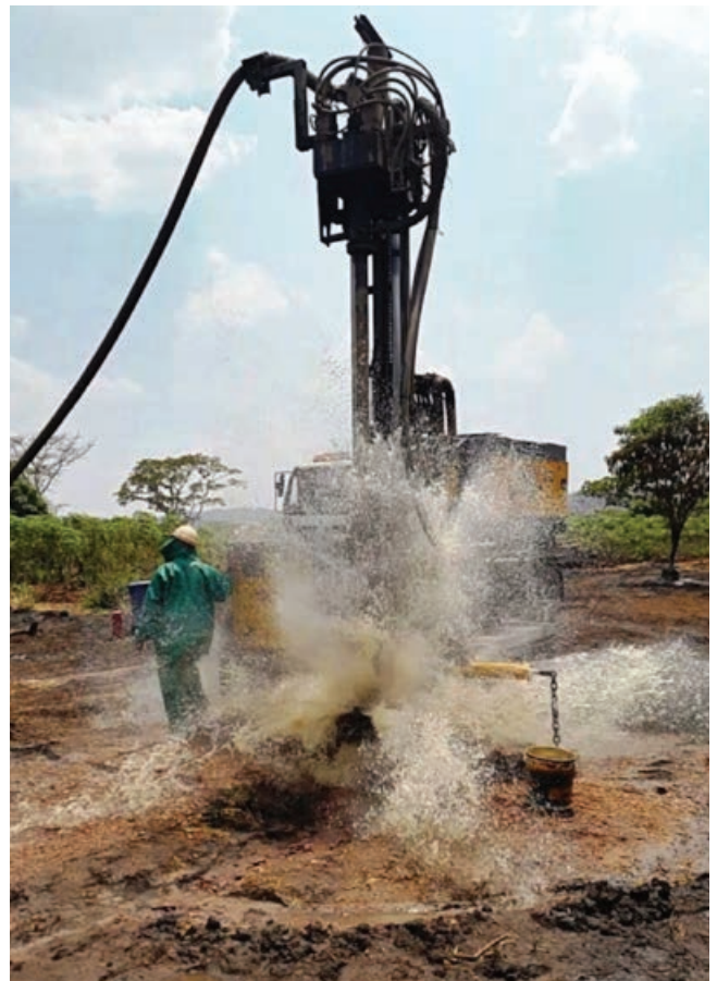
Figure 17: Water intersected in bore NWB008, September 2015.
