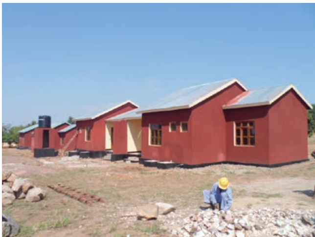
Figure 23: Duplex Ngwala school teachers' houses nearing completion in October 2014.
