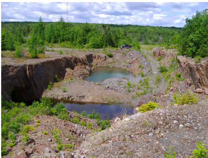
Picture notes: This small pit (looking west) was excavated in the 1980s and defines the width of the 30m-wide mineralise zone at Cochrane Hill. An underground exploration decline (portal on the left) was also developed by previous operators.
