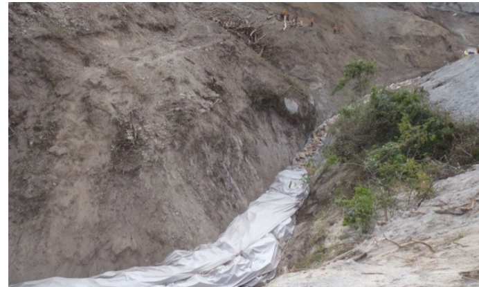
Underdrainage construction
